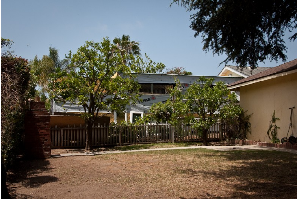
View of the new structure at 525 Alegria on 17 May from the back yard of the neighbor immediately to the east.
