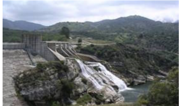
Gibraltar Reservoir is part of Santa Barbara’s water supply network.
